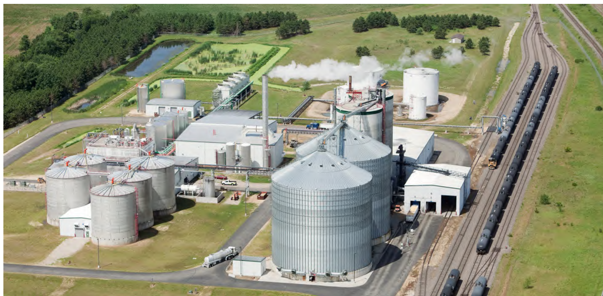
Figure 6. Aerial view of ethanol biorefinery with railcar receiving and distribution.
